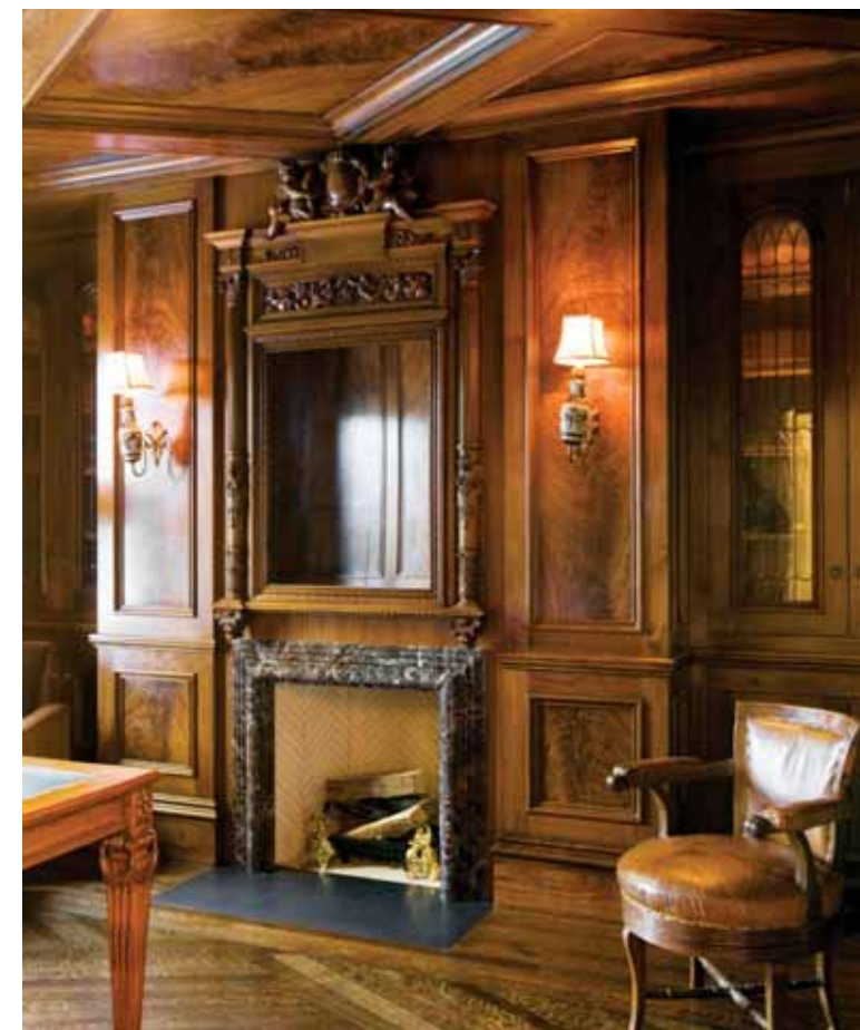
This is a high polished, semi filled lacquer finish on mahogany and crotch mahogany. A shadow glaze was used to accentuate the carved and milled details.
