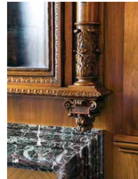
Close up of the woodcarvings, which demonstrate how adding color (shadow glazing) to the recesses and details of the carvings will accentuate those details.
